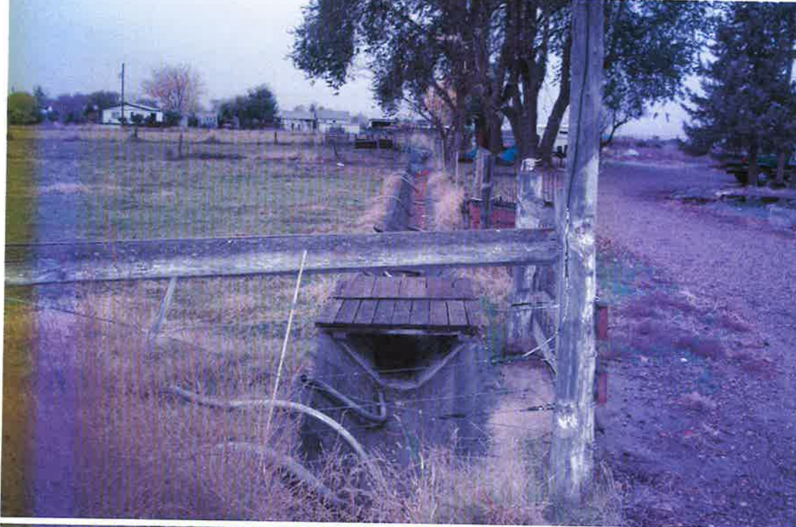
PIC#1 Cement ditch with Gravity Flow IRRIGATION (TUBES)
