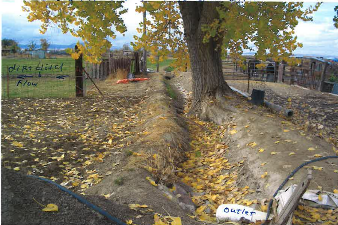
PIC#1 End of pipe FROM pump to open ditch
