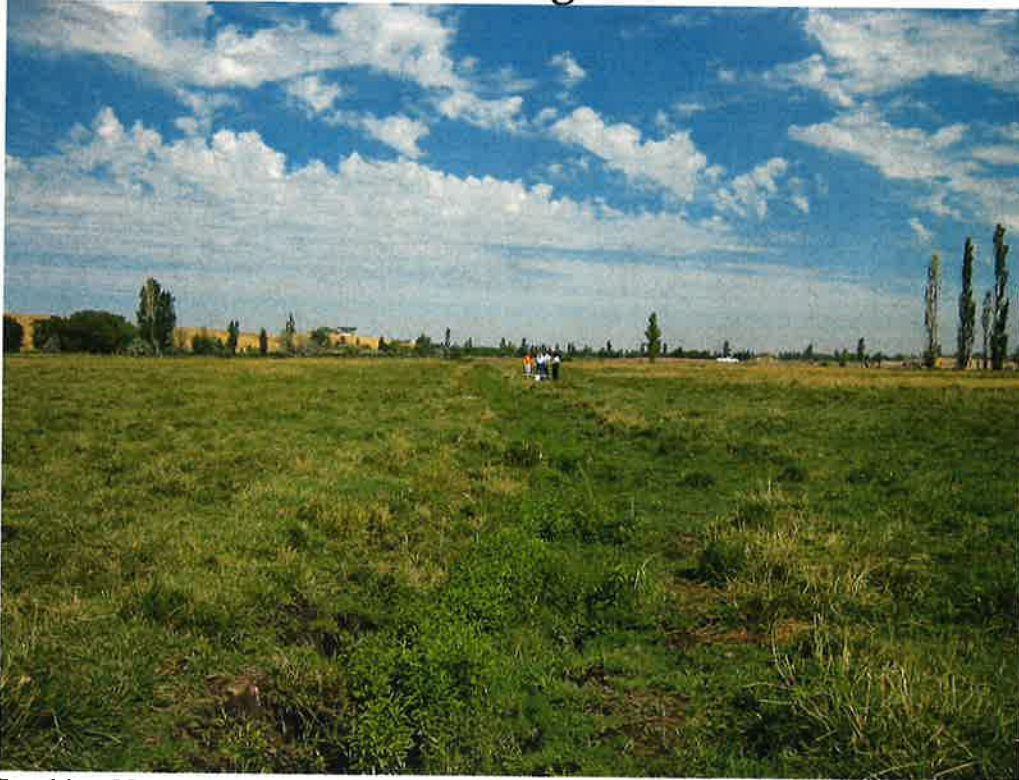
Looking North at the ditch that the Manning's calculation was done on. This is the Waste water ditch.
