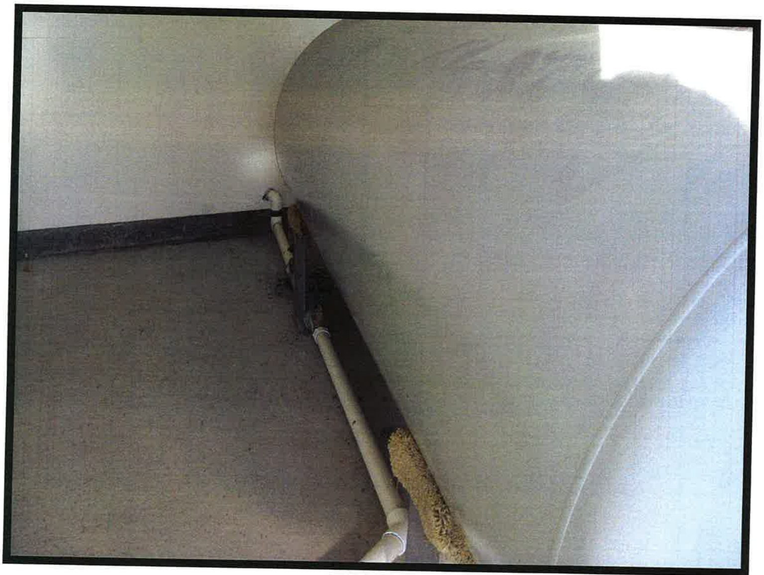
Friends Well Storage Tank
