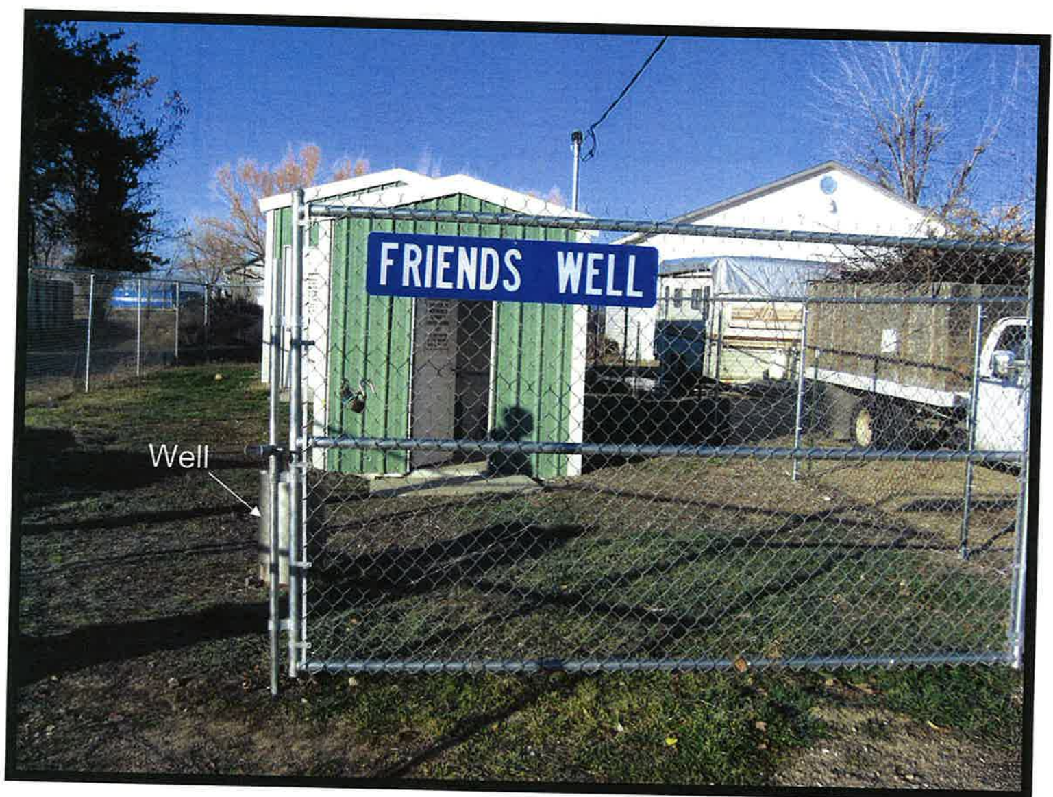
Friends Well Pump House (Storage tank in Rear Building)
