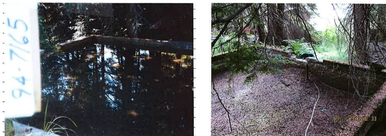
Figure 3. Photo on the left is from the Water Right Backfile. The photo on the right is the current dam/collection box on the property, at the GPS location described above.
