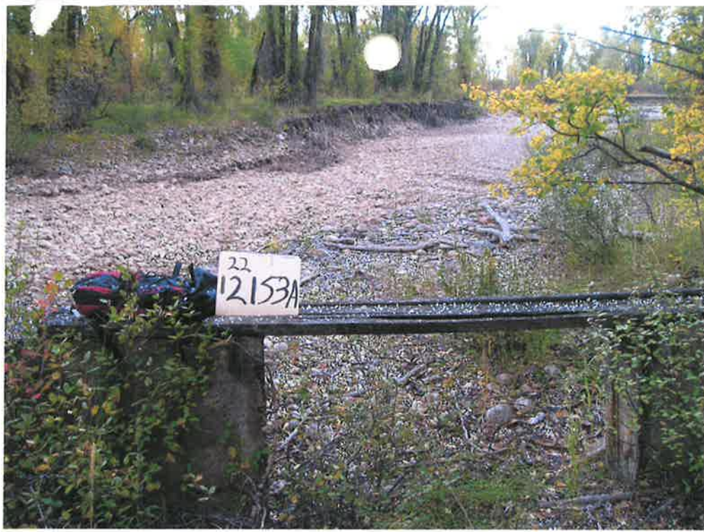
2nd picture of Gilroy's headgate on Teton Creek - tag is on headgate wall,
