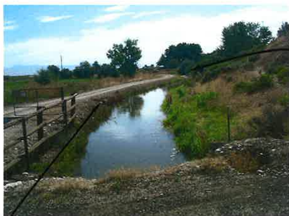
Pic 28 looking east toward the previous pan shot location. This shows where Pioneer Ditch is diverted into the Franklin Ditch system. Head gate In the very close foreground is the edge of the farmstead access road.
