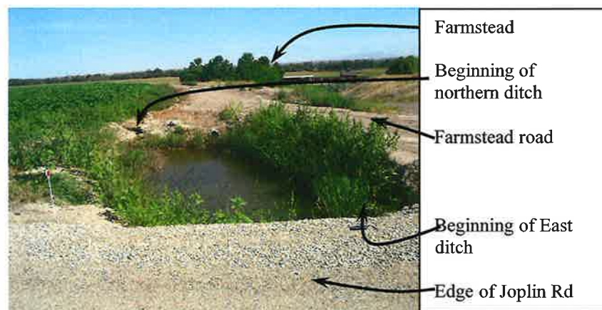
Pic 29 looking north and shows the entry location of the waste water. Water can be diverted north from this pond or east. GPS
