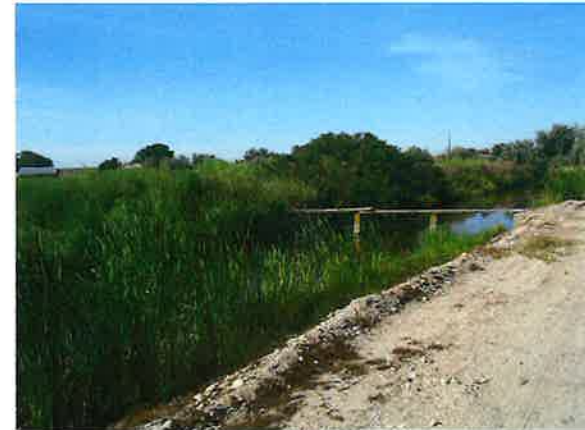
Pic 20 looking west southwest. Support structure for historic flume carrying water across the Pioneer ditch
