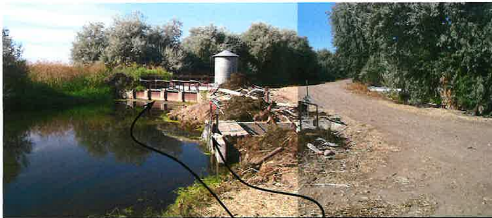
Pic 18-19 looking SW to WSW across Pioneer Ditch Diversion control structure.
