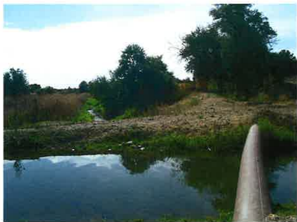
Pic 25 is looking ESE across the same flume as shown in the previous pan shot. This shows that the flume is associated with the upper or south channel at this location.
