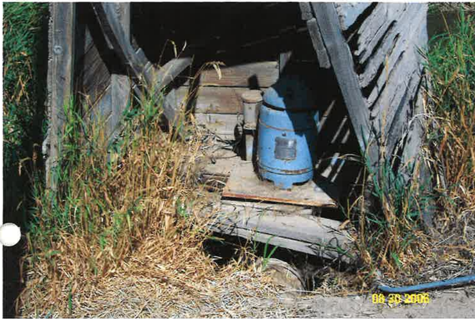
7 1/2 HP CLOSE-COUPLED TURBINE PUMP 63-5318 5318
