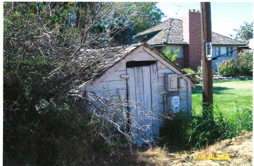
WELL HOUSE LOOKING EAST
