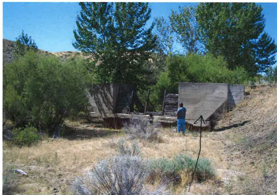
DRY CREEK DIVERSION (Abandoned)
