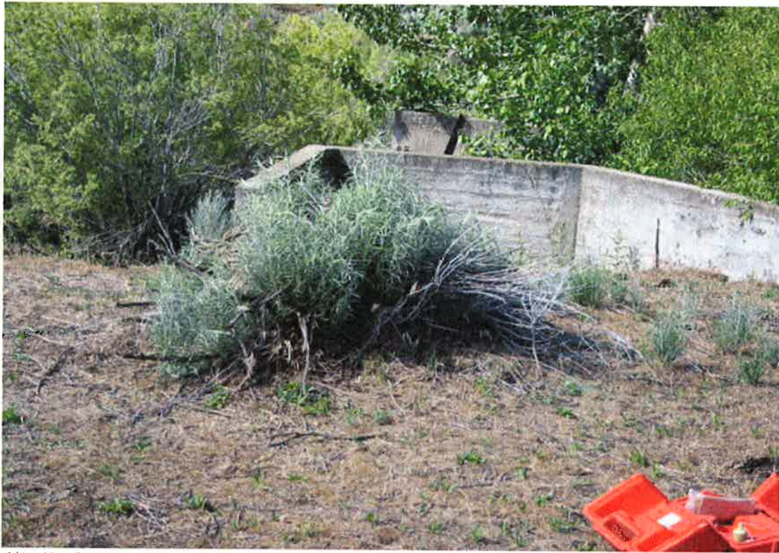
6/11/07 [IMG_0095.JPG] – T4N R2E S4 SESW. 6-11-07 – SESW S4, T4N, R2E - top photo looking down at concrete diversion dam. Top of dam nearly at land surface.
