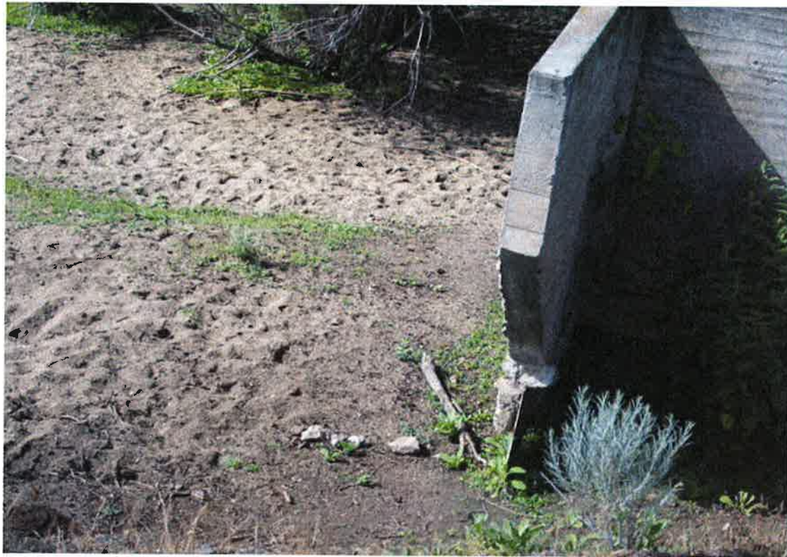
6-11-07 – [IMG_0096.JPG] - SESW S4, T4N, R2E - from land surface looking down at dry Dry Creek bed and dam.
