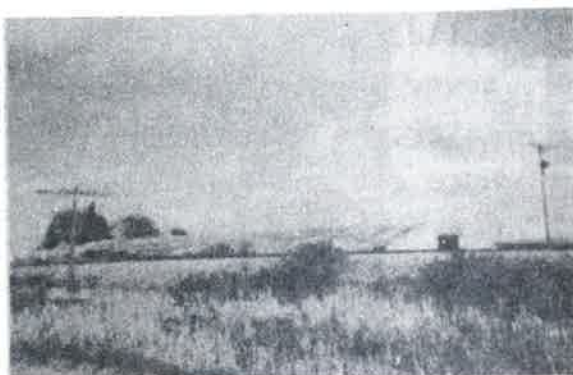
The Wilcox potato storage cellar. Picture taken over the train tracks.
