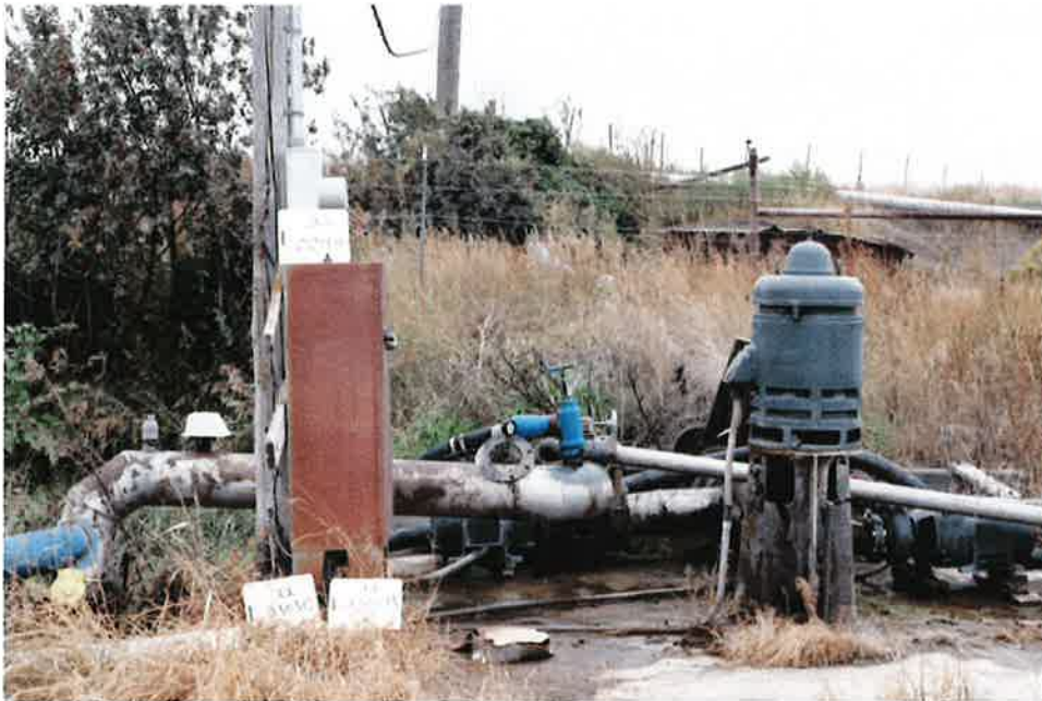
Photo #1, POD looking south east.
