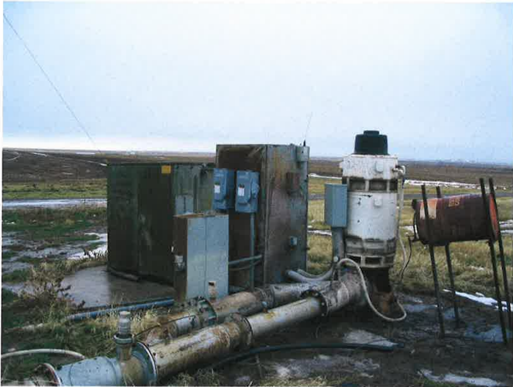
A22-7048, Looking West
