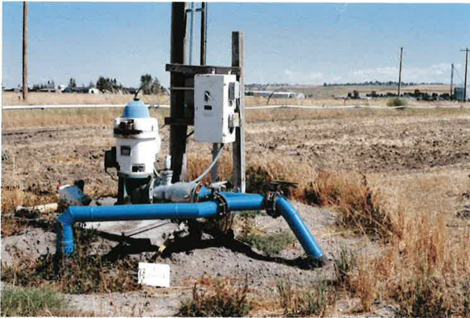
Photo #1, POD looking north east.
