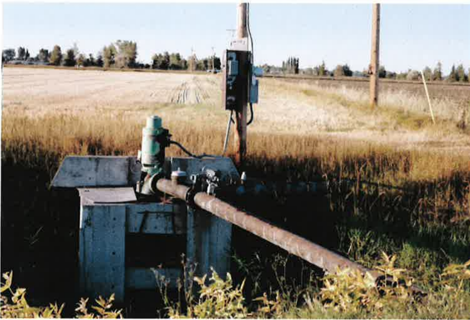
Photo #1, East POD looking south.
