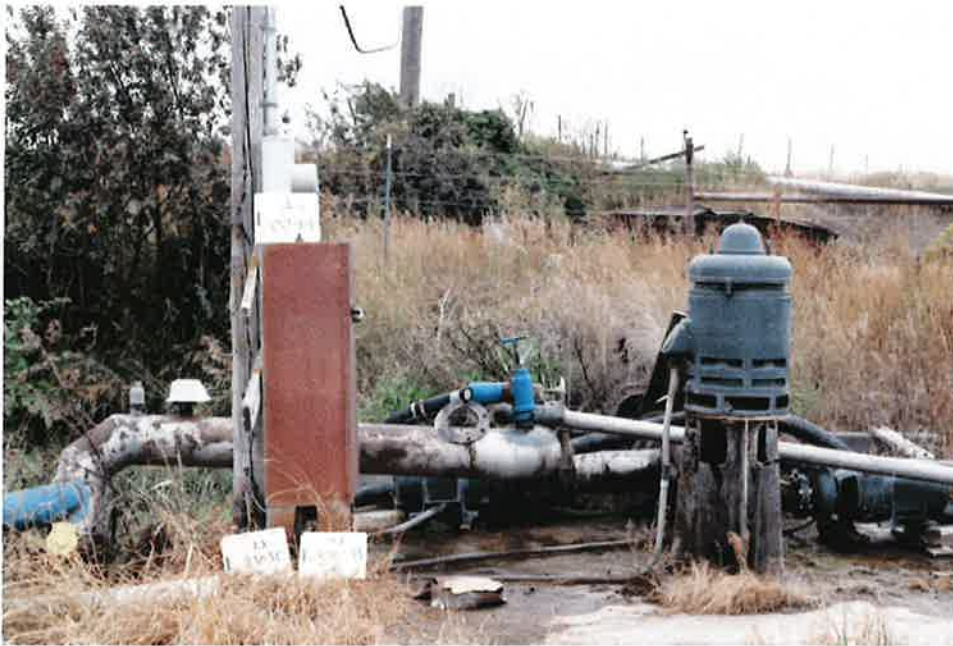
Photo #1, POD looking south east.
