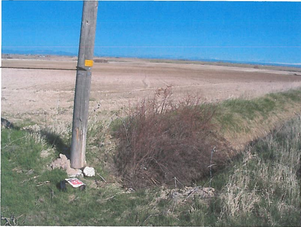
A22-2145, wastewater pick-up ditch
