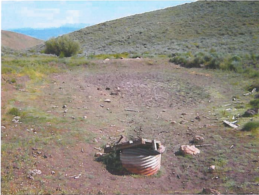
Culvert spring box and reservoir. A stock tank below the reservoir catches overflow. The stock tank is not visible in the picture.
