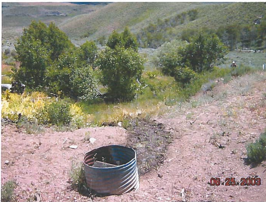
Good Spring and culvert spring box. The spring box fills a stock tank below.
