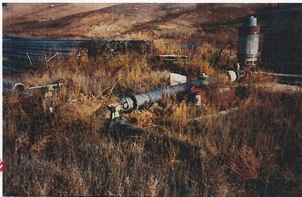
PHOTO TWO- View northeast of well No. 1. 'T' section shown in foreground.
