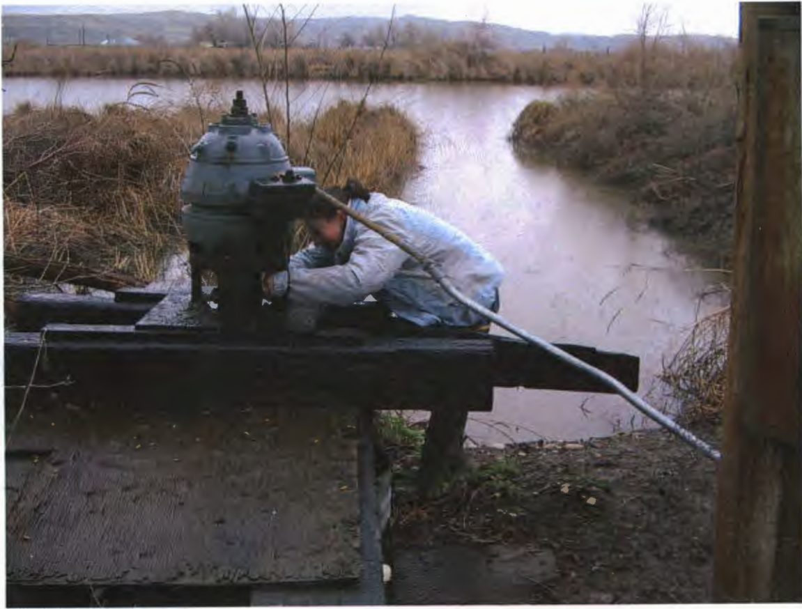
67-4012 POD, picture taken looking toward Buttermilk Slough
