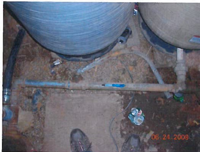
Figure 1. Owyhee Motorcycle Club Diversion Works
