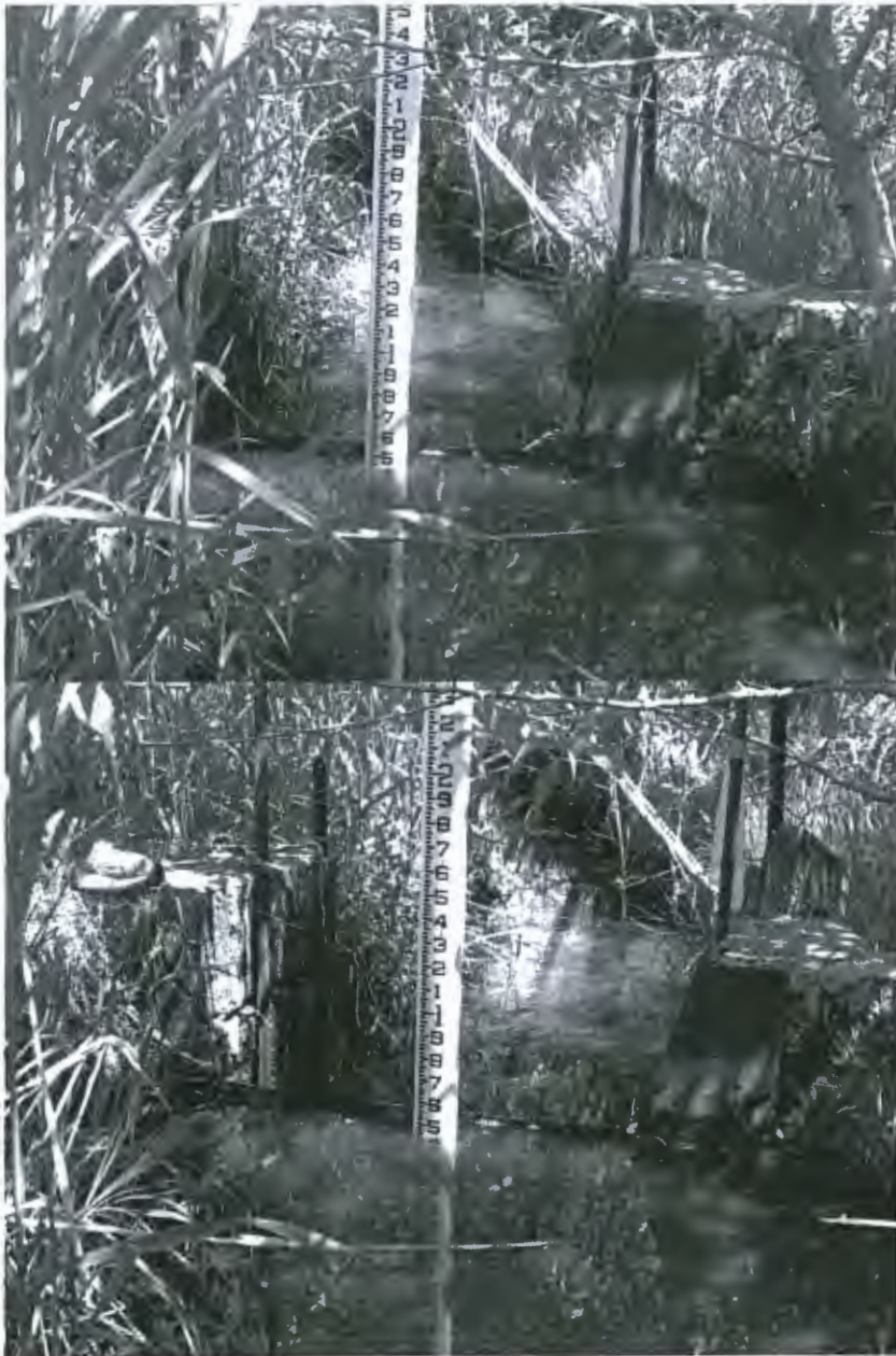
Above photos are taken of Ridenour Weir from just upstream. Rod instream is for scale. Actual measurements are in file 67-4052D.
