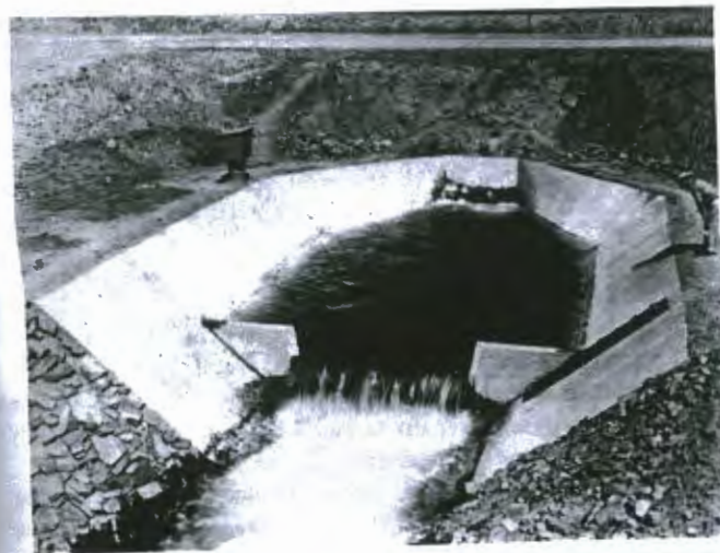
Figure 7.—Cipolletti weir with a well-type head-measuring station. PX-D-53011.
