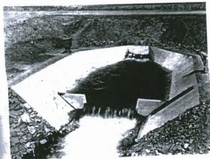
Figure 7.—Cipolletti weir with a well-type head-measuring station. PX-D-53011.
