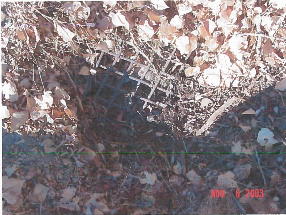
POD #2 Catch drain to collect wastewater across road from house.
