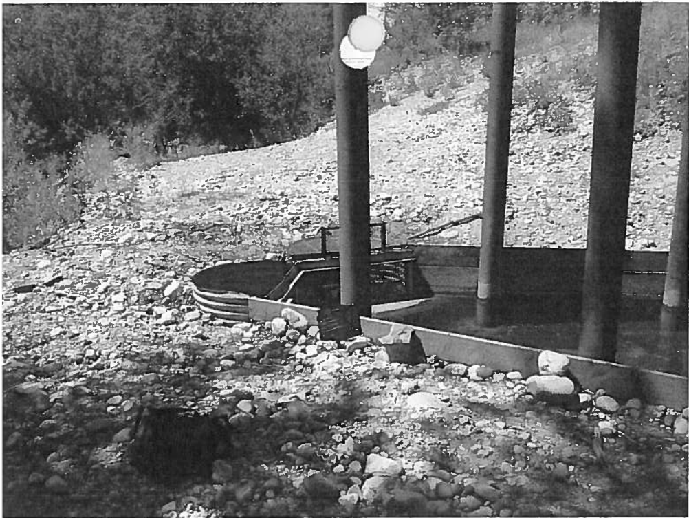
Killpack headgate - Wyoming diversion Boyd Smith and others use this headgate.
