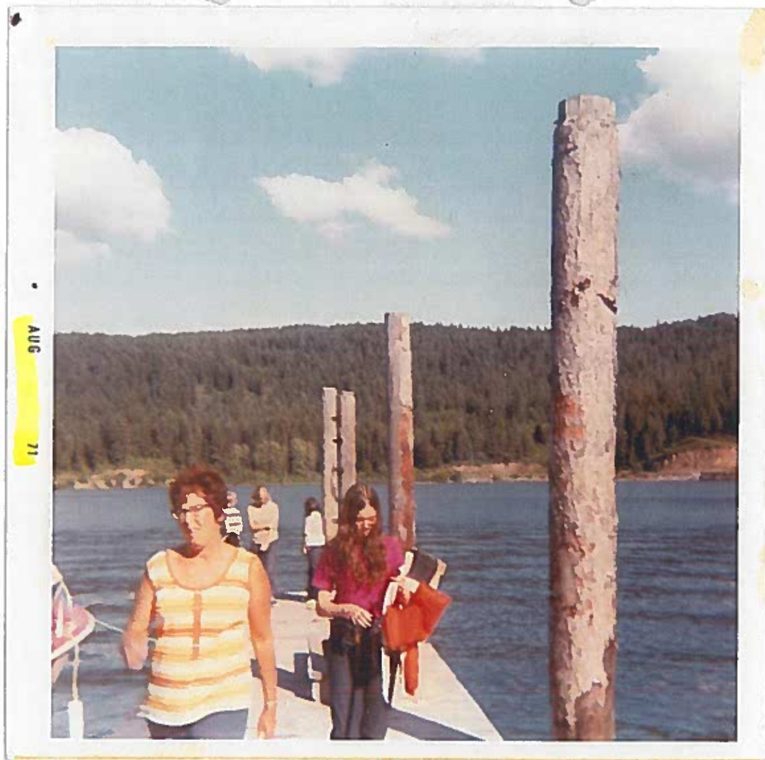
Aug 1971 - Dock with Pilings at place of use (Also used to secure lake water system - Foot Valve at end of Dock)
