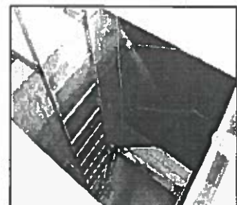
Fig. 12a – access ladder
