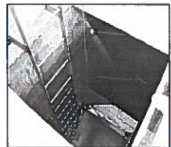
Fig. 12a – access ladder
