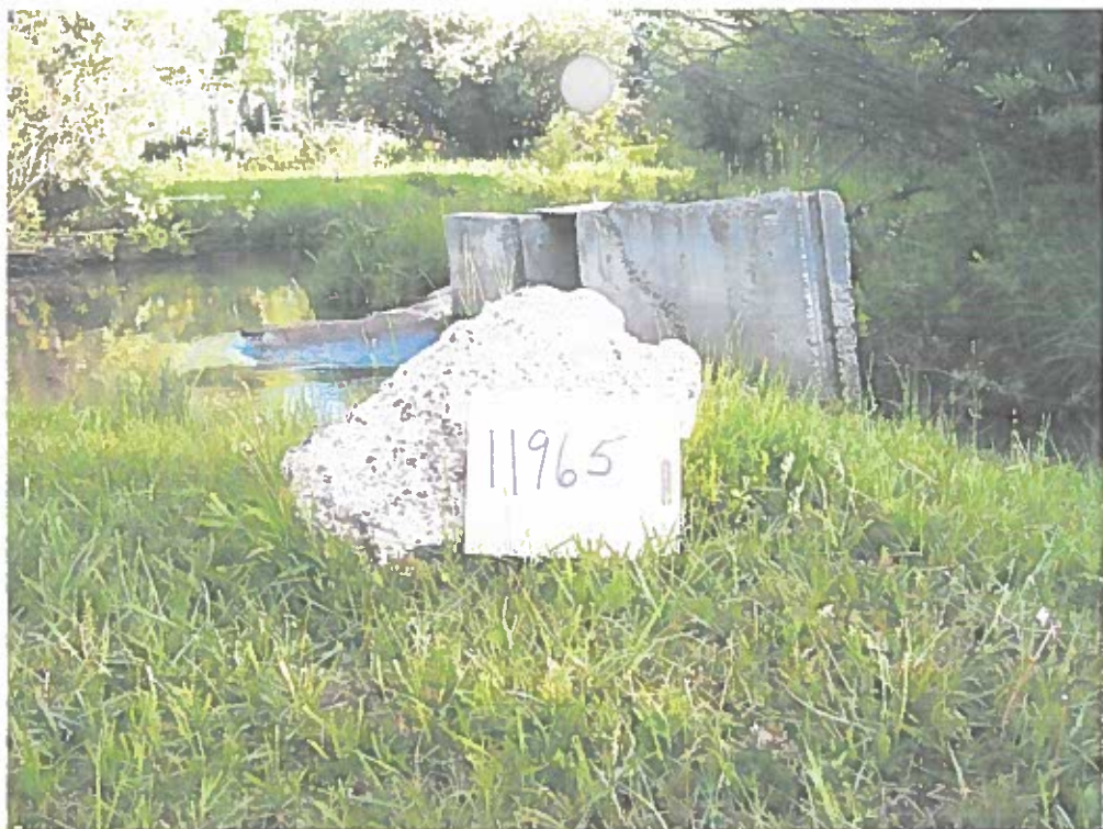
Alvie Christensen diversion out of Darby Creek
