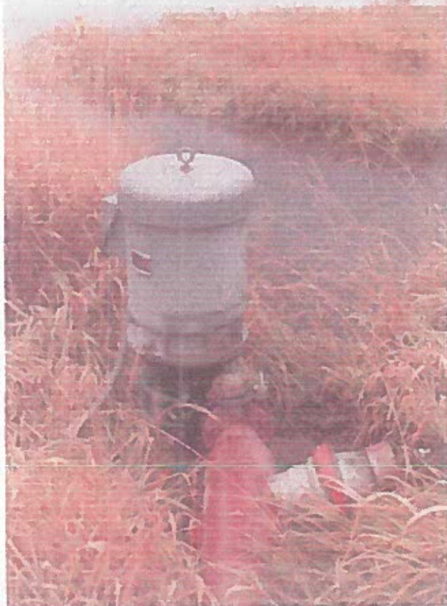
NEW POINT OF DIVERSION Marathon Motor 50hp Type TDR-BHPZ
