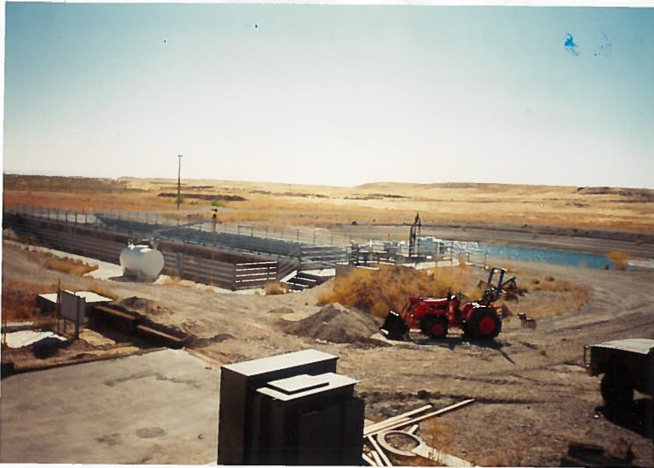
Photo # 9 10-1-96 Looking NE From the NENE of Sec 35 showing the washing water recycling facility on the left and one of 2 of the recycled wash water holding ponds.
