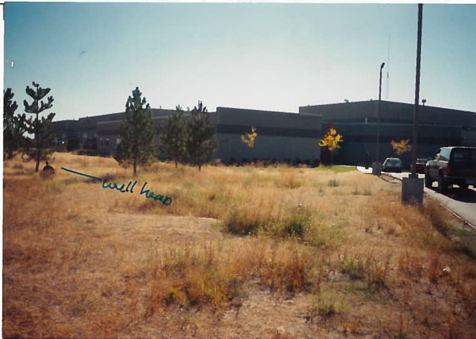
Photo #6 10-1-96 Looking NE from the NW NENE corner of Sec 35 T1S R3E showing the MATES facility and Well head. POD #1
