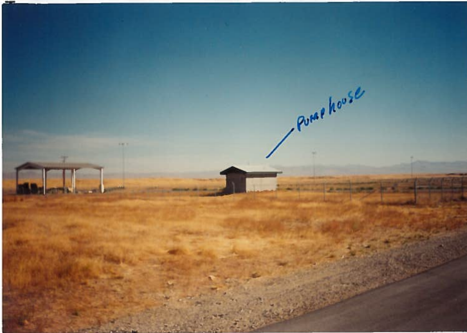
Photo #3 Looking NE from the NWNE of Sec 2 showing the ASP facility pump house and the Place of use. POD #2 10-1-96 ASP Facility
