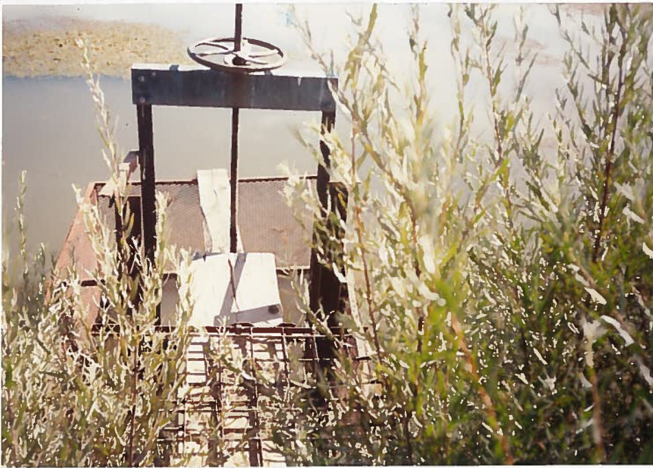
Photo #3 Looking E, From 4S 7E sec 8 SESE showing Flow control gates to outlet from Reservoir 9-4-96
