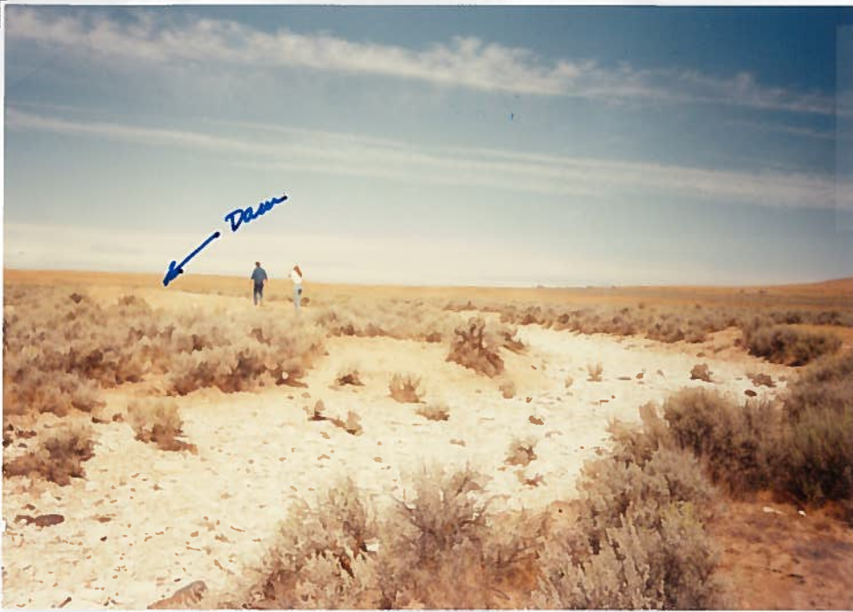
LOOKING N. FROM 45 7E Sec 4 NW 1/4 at spillway That goes around the SE End of the Dam, Photo #8
