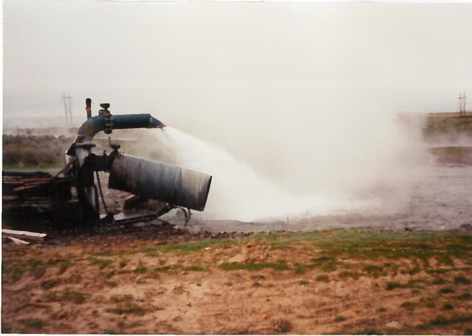
#22 P/R - Artesian well in NWSE, S1, 4S, 8E
