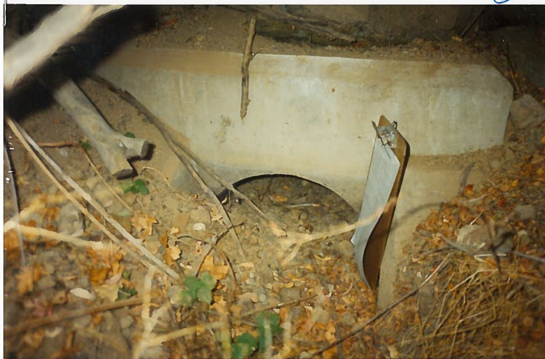
② Close-up of culvert on south side of highway. Clipboard is 13 inches long.
