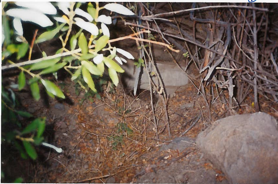
① Culvert on south side of highway
