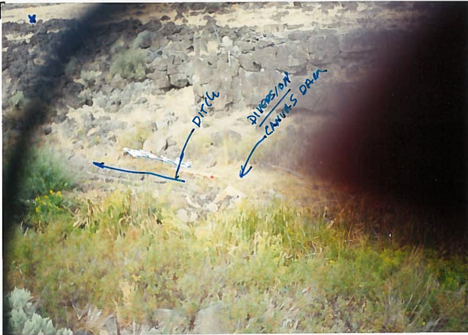
Photo #9 9-18-96 Looking North from the NW SW corner of Section 2 showing the canvas dams used to divert water from Rattlesnake Creek into a ditch going west to the POB,
