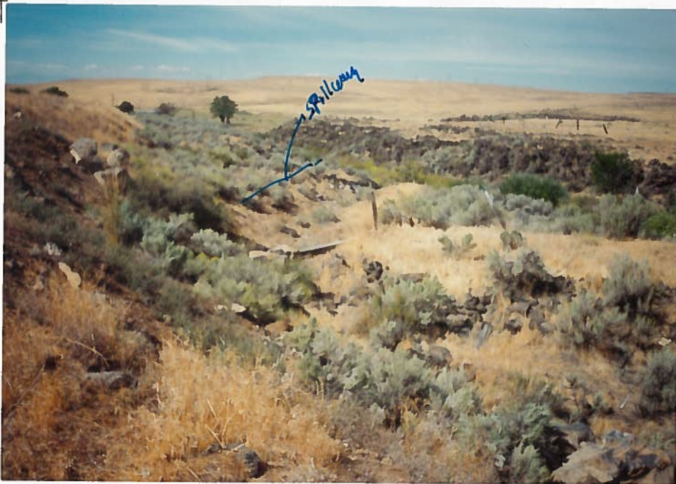
Photo #6 9-18-96 Looking NW from the NW SW corner of Section 2. Showing spillway in former dam, along Rattlesnake Creek
