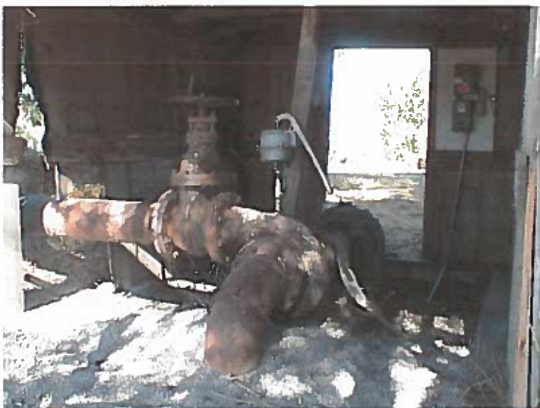
Old well house near concrete pad shown above (not used).
