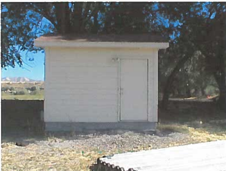
Deep well pump house
