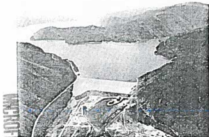
Palisades Dam and Reservoir
