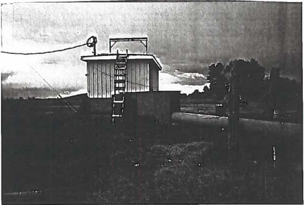
Filter-Parshall Flume & Mixing Shed
