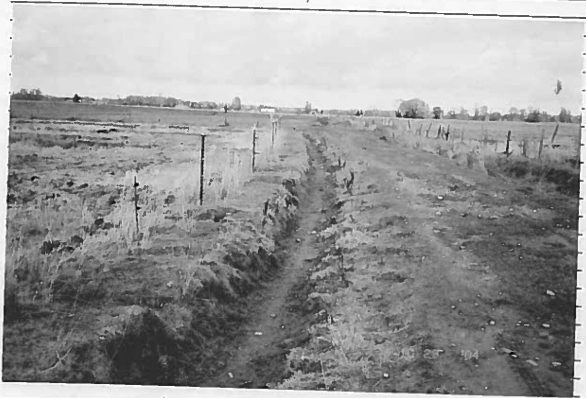
Photo showing Rocky nature of ditches.
