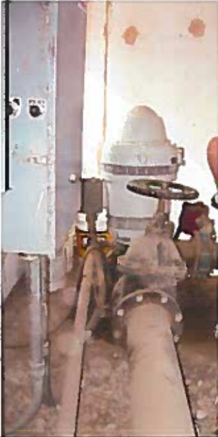
This photo shows the well located just west of the office and packing plant.
