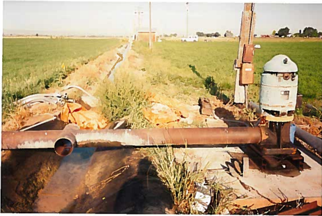
#1 PID and concrete delivery ditch looking West from well site toward P14.
