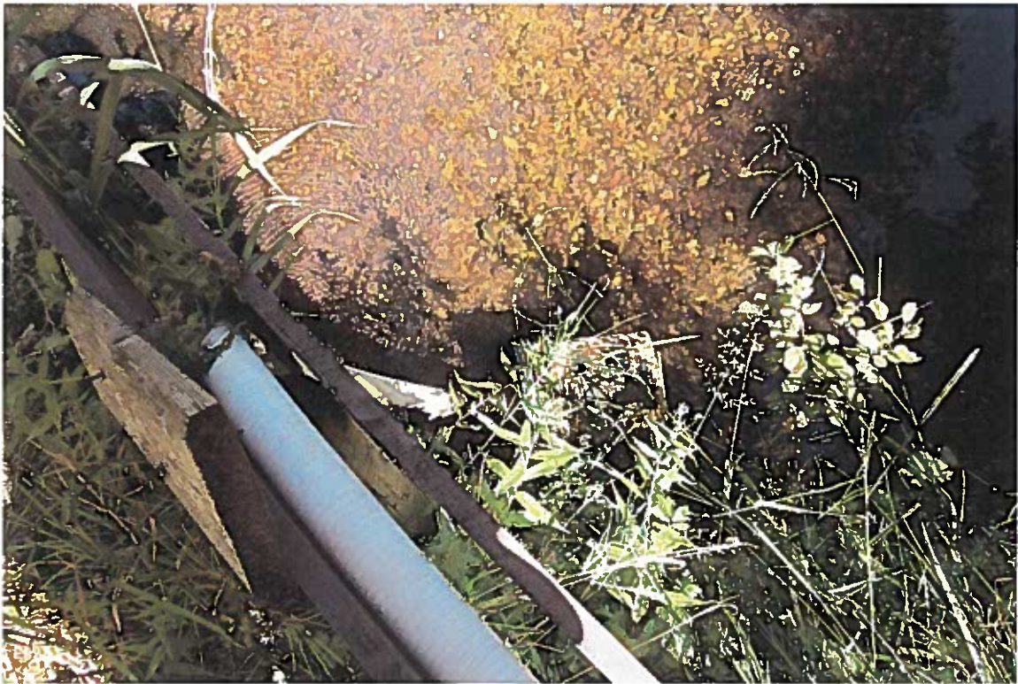
Diversion from Sage Creek in NENW S. 36 T53N R3W
