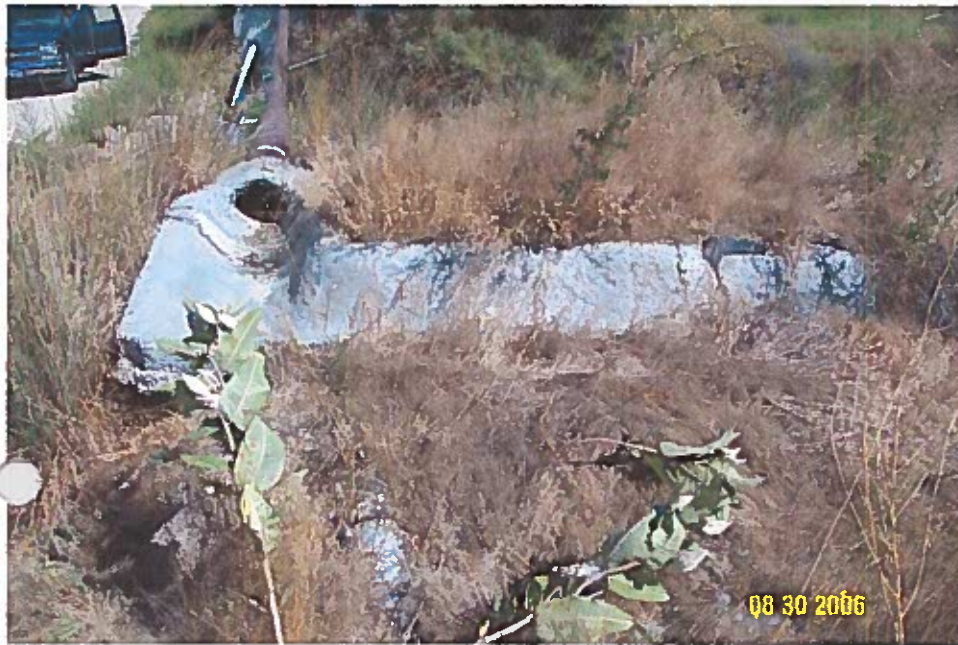
OUTLET STRUCTURE SOUTH SIDE OF DRAIN LOOKING NORTH
