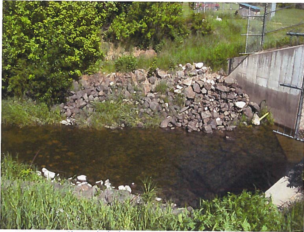
Photo 11 (06/06/2013) - Right Downstream Groin Area
