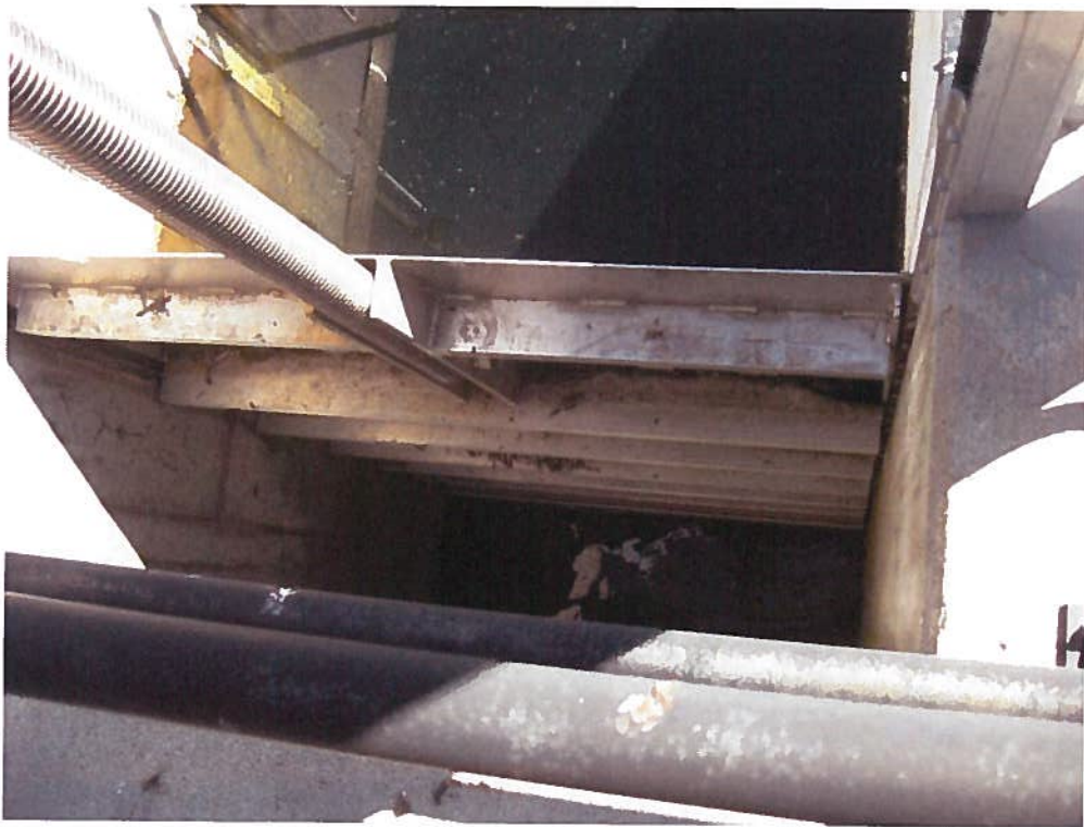
Photo 8 (06/06/2013) - Right Gate Closed
