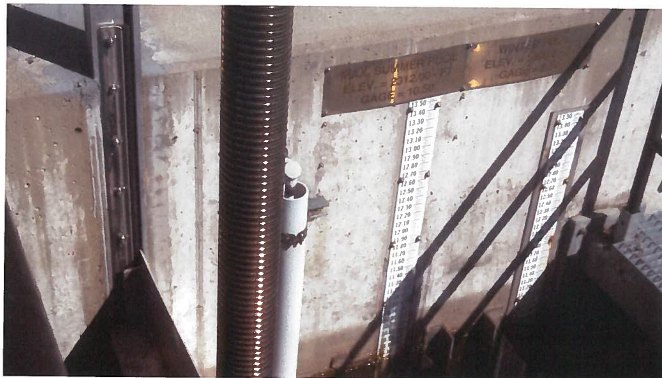
Photo 2 (06/06/2013) - Staff Gages and Stage Signage
