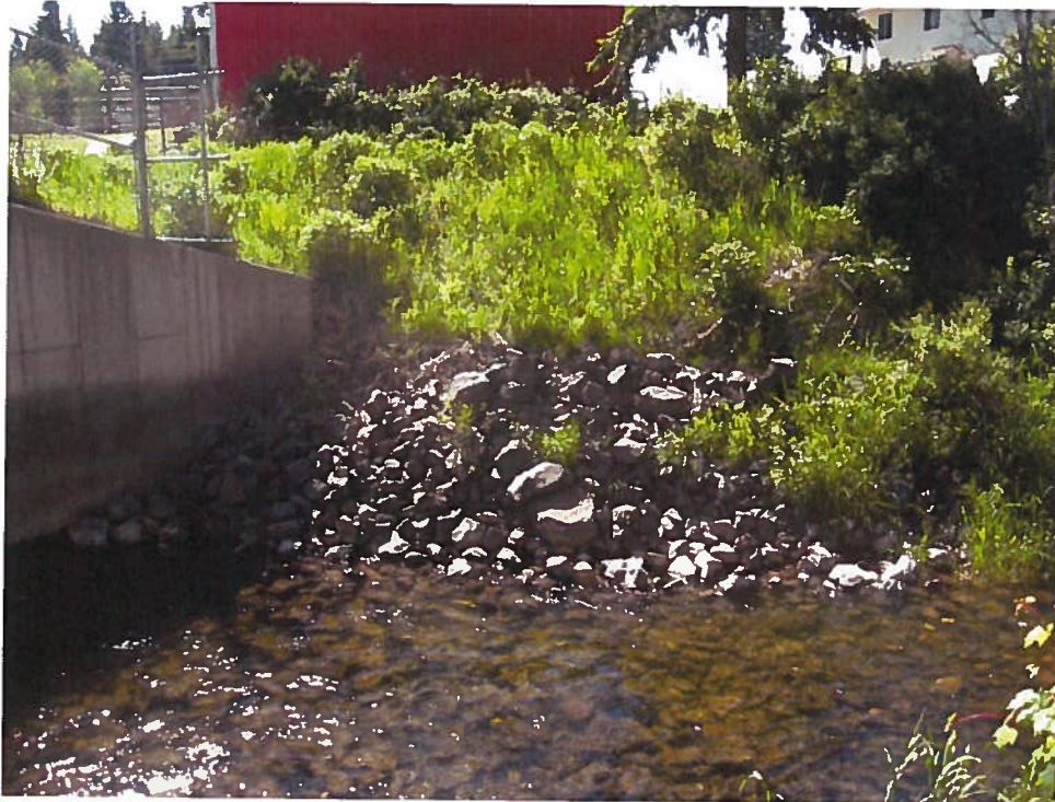
Photo 12(06/06/2013) -Left Downstream Groin Area
