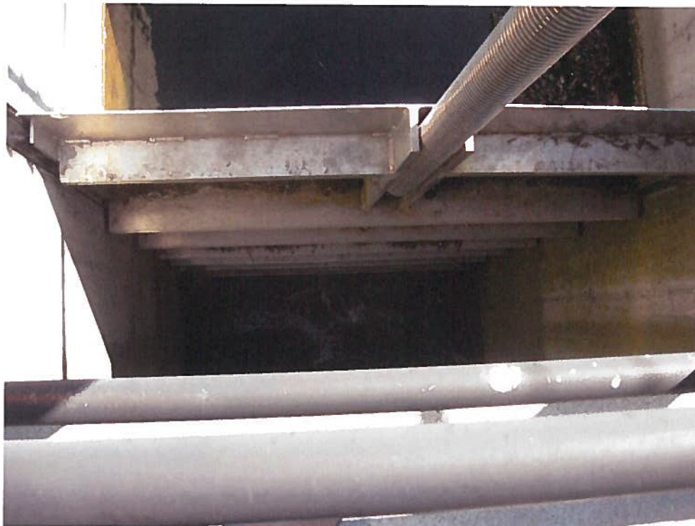
Photo 9 (06/06/2013) - Left Gate Open, Note Flow at Base
