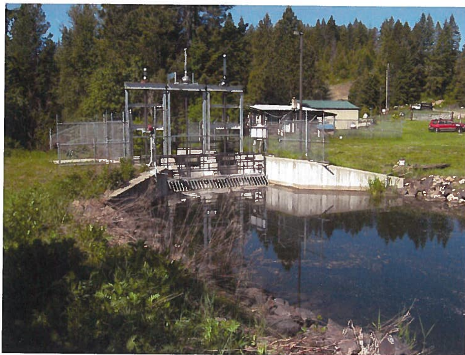
Photo 1 (06/06/2013) - Overview of Dam and Facility
