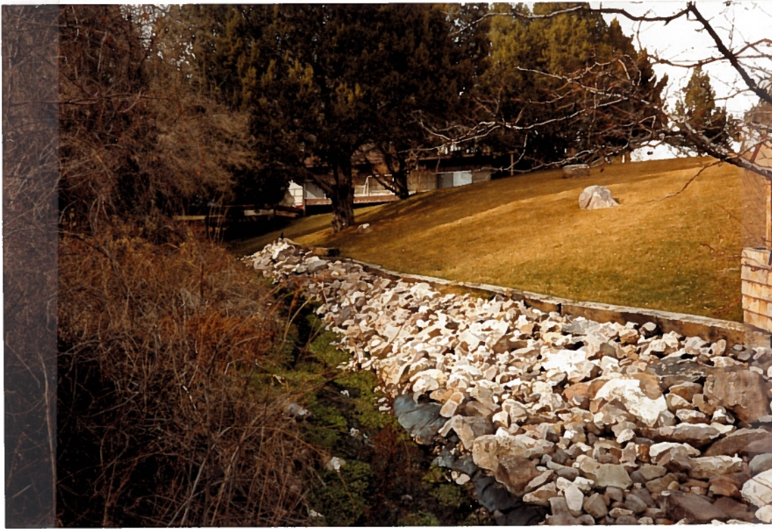
Looking N.W. from a point near the S.E. corner of the Collins property.
