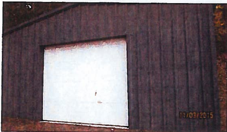
LOOKING EAST AT DECONTAMINATION UNIT JUST NORTH OF HOSPITAL FACILITY.
