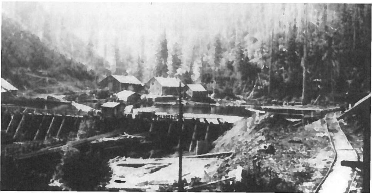
View of Camp 3, dam and head of flume from below the dam, 1929 Photo courtesy of Lew Stearns
