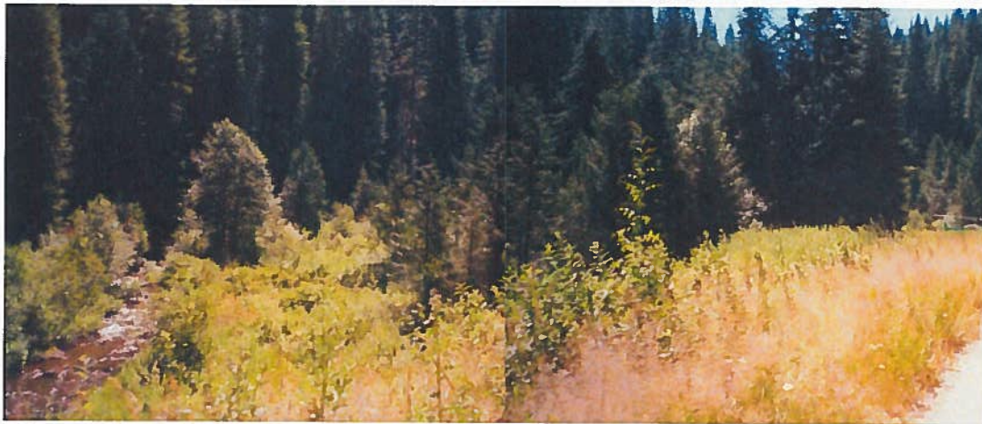
Looking upstream site of Camp 3 dam and head of flume, 2000 Road in lower right corner is approximately the same location as railroad in 1929 photo.
