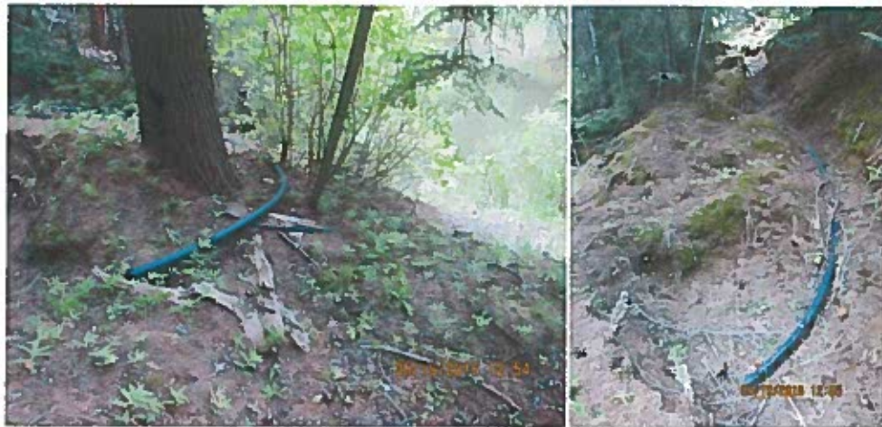
Large water line running from pond through trench up hill
