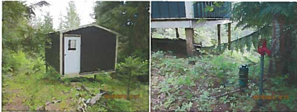
Cabin B – 2" PVC pipe stub under corner of home and water spigot with control valve next to the home.
