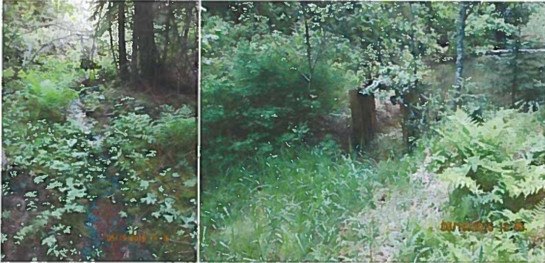
Seepage from toe of dam (pond 1 on map) flows down draw into lower pond (pond 2 on map)
