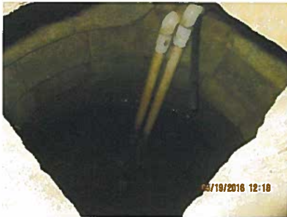
Black plastic conduit into cistern and out the pumphouse
